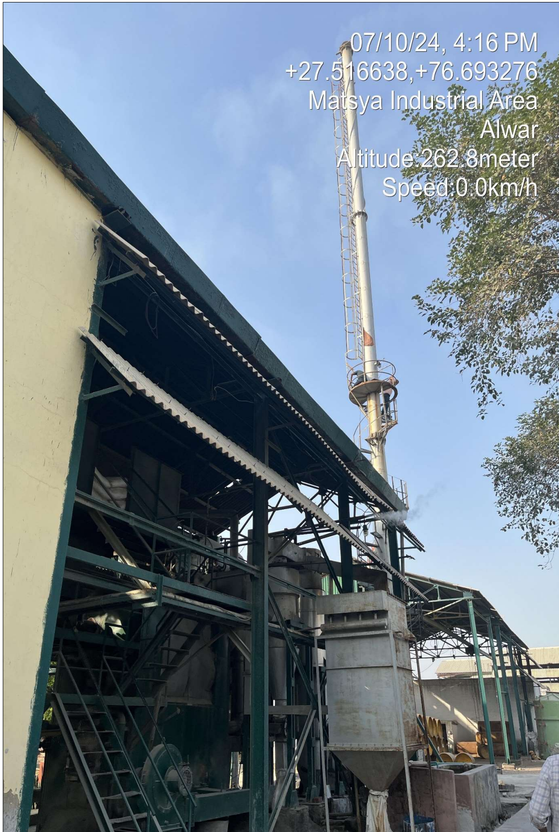
Fig 04: Emission control measures and stack of height approx. 30 meters have been provided at the boiler installed in M/s KSJN Chemicals Pvt. Ltd.
